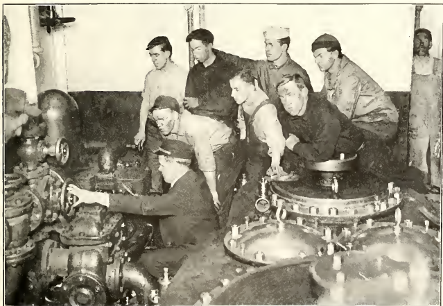
PRACTICAL INSTRUCTION IN THE BOILER ROOM ON BOARD A SHIPPING BOARD TRAINING SHIP
